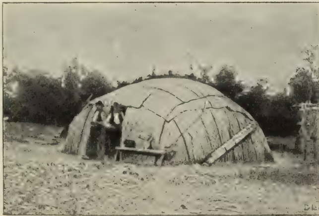
CHIPPEWA BARK HOUSE. (GILFILLAN)
